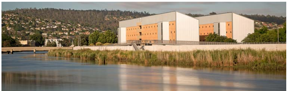
The University of Tasmania's new student accommodation complex in Launceston.
