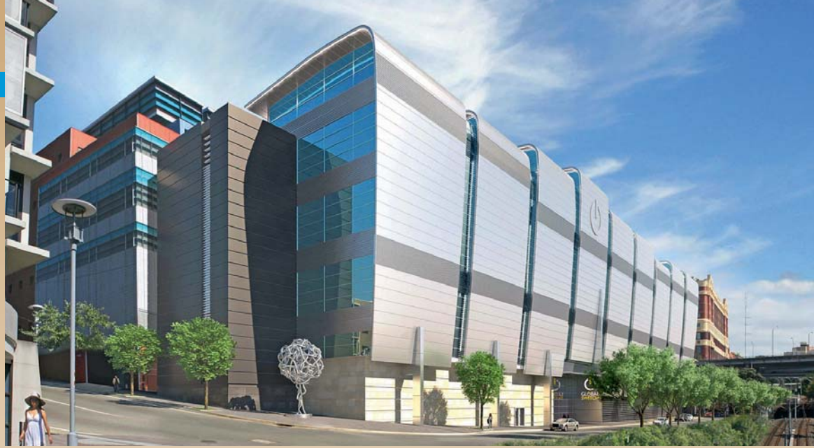
Global Switch's expanded Sydney East Data Centre has been designed to meet its customers' requirements for the next 20 years.
